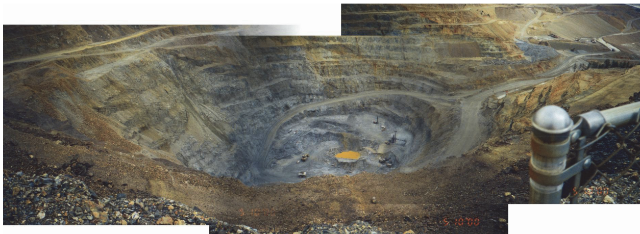
Figure 1. Acid drainage collecting in the pit bottom sump at Golden Sunlight Mine. Note the orange colour of the water in the pit sump, indicative of the acid water draining into the pit.
