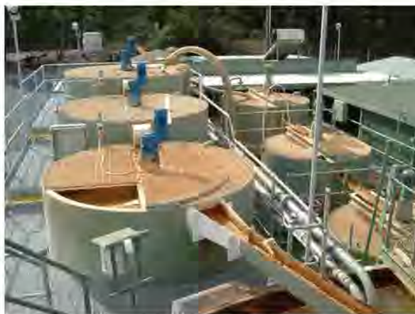
Figure 7. New treatment plant showing second parallel series of reaction vessels (upper left) with existing upgraded plant (lower right).
