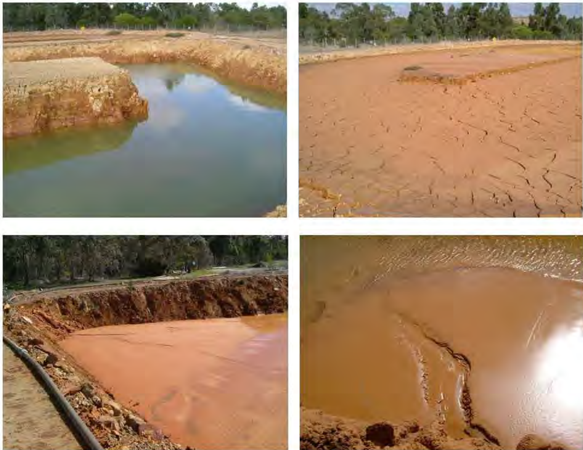
Figure 8. Sludge pond. Low-density sludge prior to plant upgrade partly fills one of the two sludge ponds (upper left). Sludge pond full of partially air dried sludge prior to desludging (upper right). High-density sludge entering the sludge pond after plant upgrade (lower left and right).
