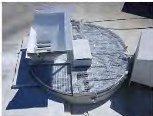
Figure 5. Below ground hydrated lime storage, mixing and dosing system.
