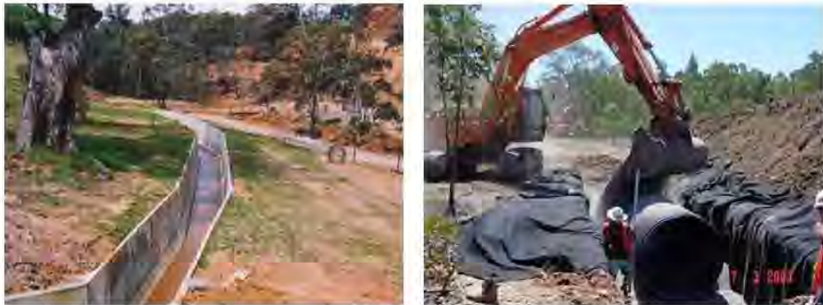
Figure 2. Dawesley Creek diversion drain. Laying pipe for the underground segments of the drain (right) and open channels (left).
